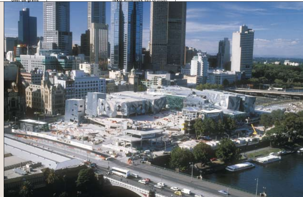
Foto rechts Federation Square, 2002, Melbourne, Victoria, Australia. Architect: Lab architecture studio in association with Bates Smart. The city's financial district rises behind the new cultural precinct.
