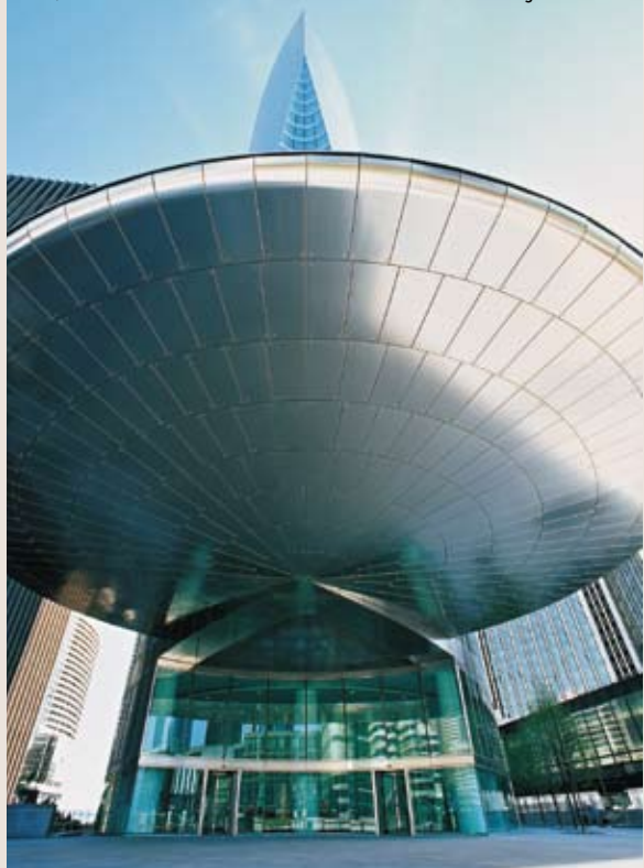
Foto links EDF Tower, 2001, Paris, France. Architect: Pei Cobb Freed & Partners Architects. The tower, reflected in one of the water features of the landscaped public plaza.
